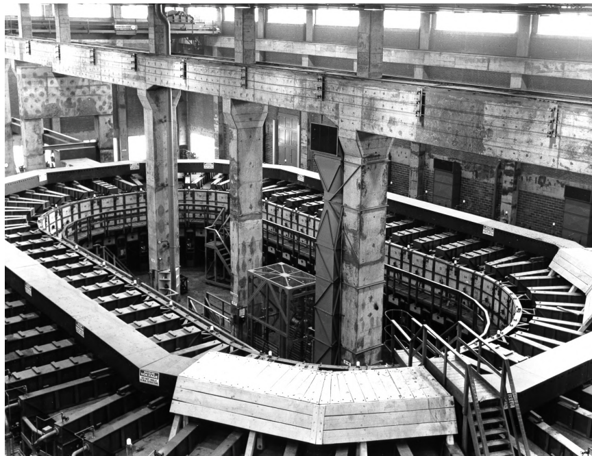
Figure 3.2: Calutron alpha “racetrack.” Y-12 facility, 1944. [275].
